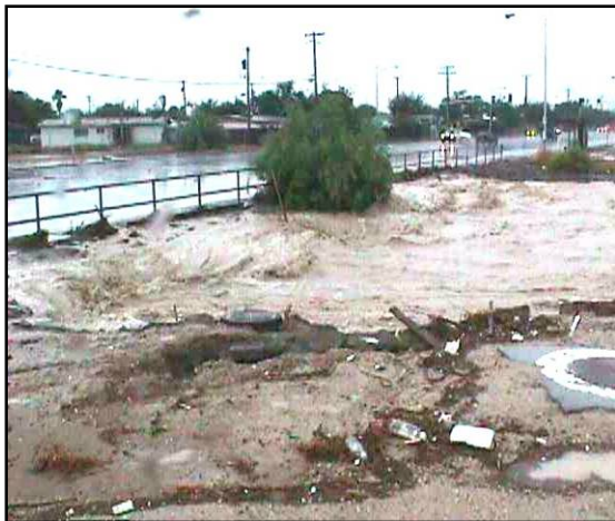
Photo 1 Subsurface Currents Upstream of Submerged Culvert
